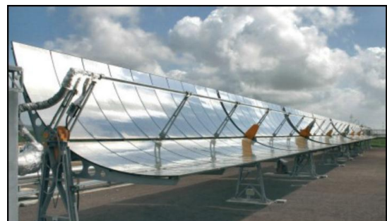
Figure-2: CSP Parabolic Trough Solar Collectors [1]
