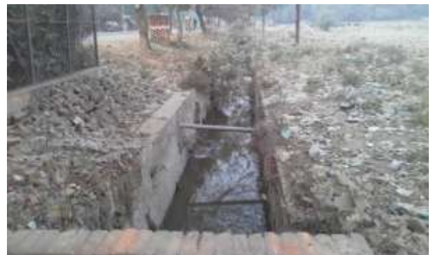
Open drain on the site periphery
