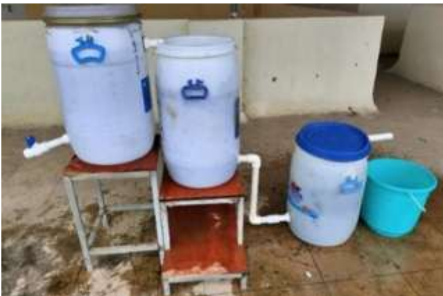
Image 1 : Image of Filtration Treatment Unit
