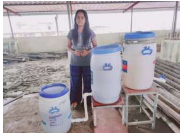
Image 2 : Filtration Treatment Unit
