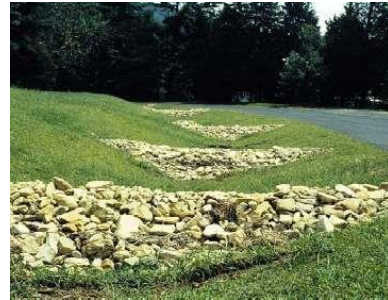
Figure 3: Grass Swales Source:(Virginia Stormwater Management Program (VSMP), n.d.)
