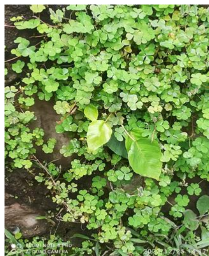
Location- Old Building State Bank of India Sidhi
