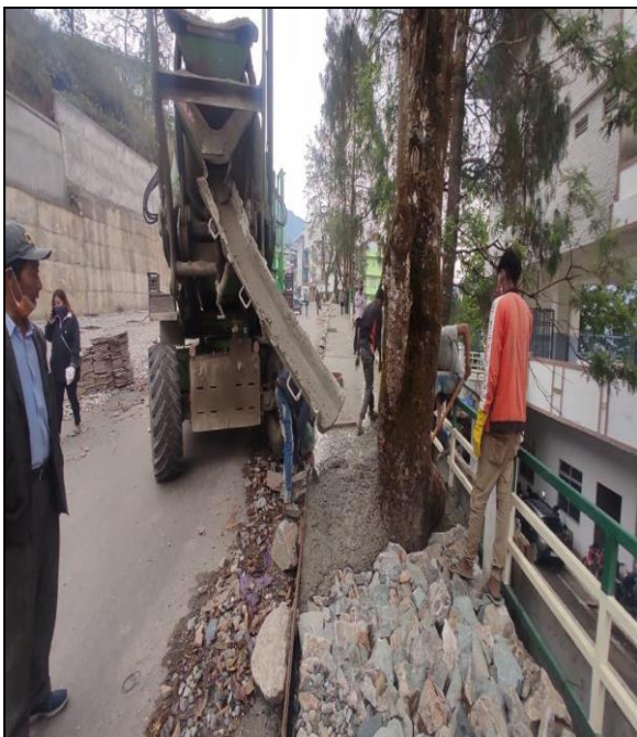
Figure 11: Working of CRSM wall casting using manpower & TM
