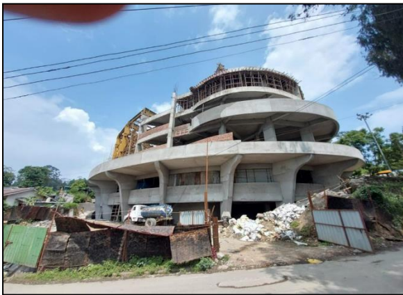
Figure 20: Angular view of the structure
