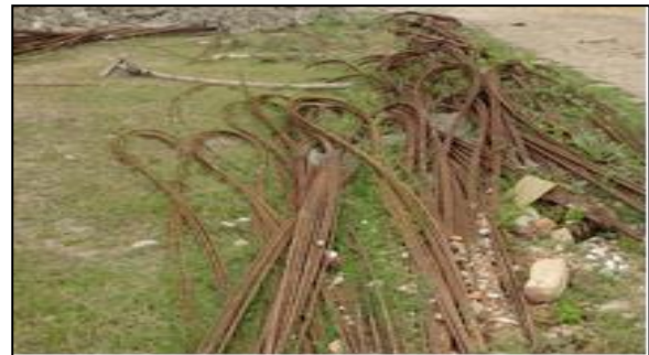
Figure 6: Rusting of iron at site from long time
