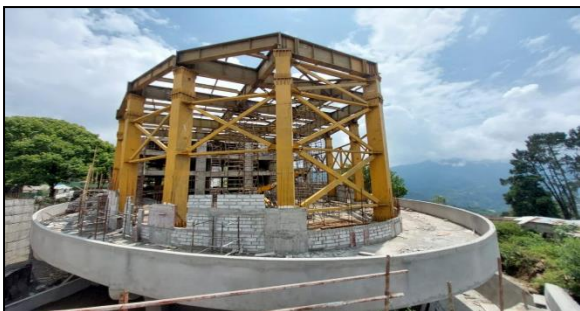
Figure 22: Top view of the structure
