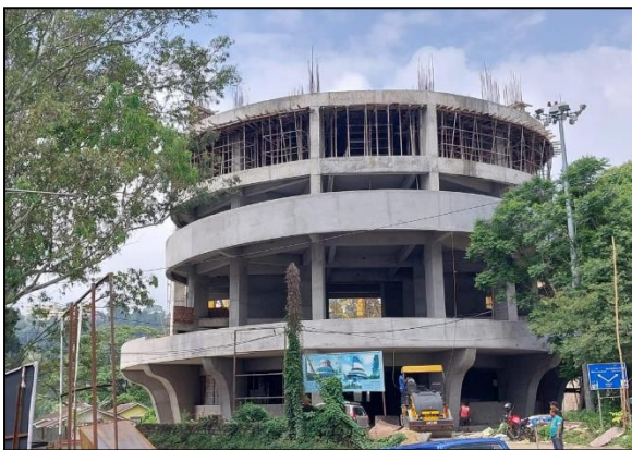
Figure 21: Front view of the structure
