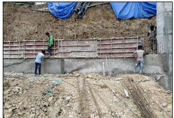
Figure 14: Shuttering work going on for RCC retaining wall
