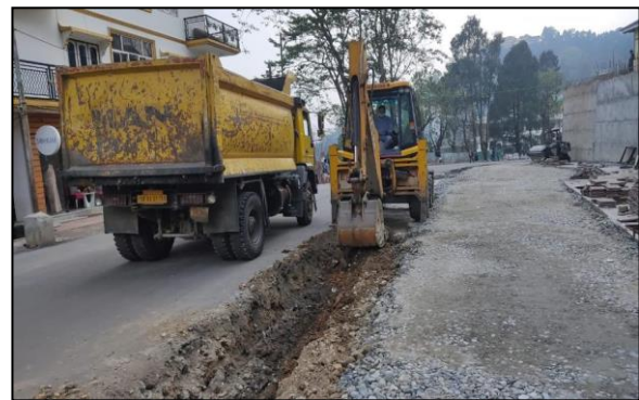
Figure 9: Work is going on under this circumstances using JCB & Mini Tata
