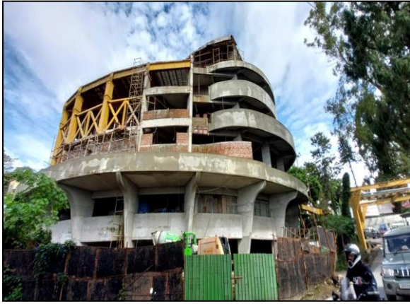
Figure 19: Back View of the structure
