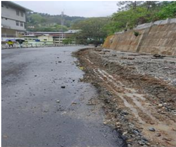
Figure 3: Excavation work due to water passing for transportation
