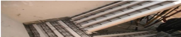
Figure 9: Stair case construction
