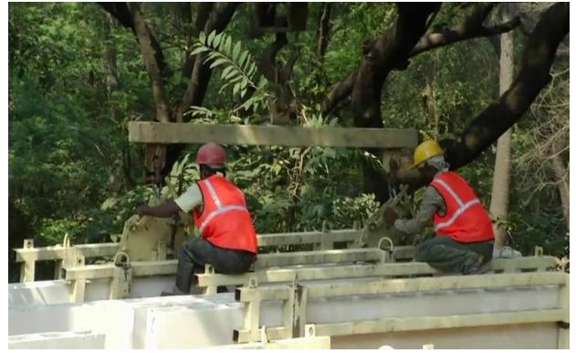
Figure 5: Transportation and lifting of the GFRG panel
