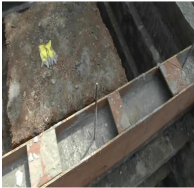
Figure 6: Foundation part of the construction
