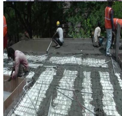
Figure 8: Roof slab construction
