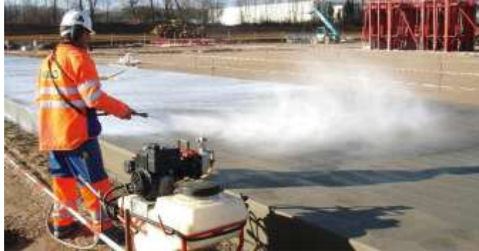
Fig 1.1: Curing should begin as soon as the concrete stiffens enough to prevent marring or erosion of the surface.
