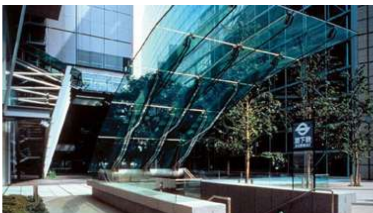
Figure 2. Glass cantilever in Yurakucho station canopy
