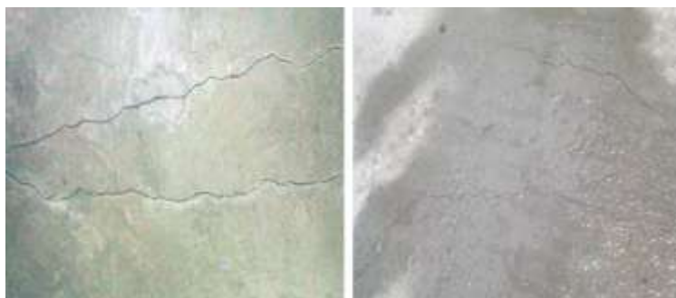
Development of cracks due to incompleteness of hydration cycle and self-desiccation (b) Poorly segmented capillaries
