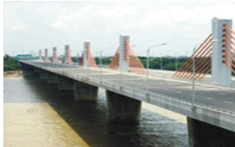
The Extradosed Bridge
