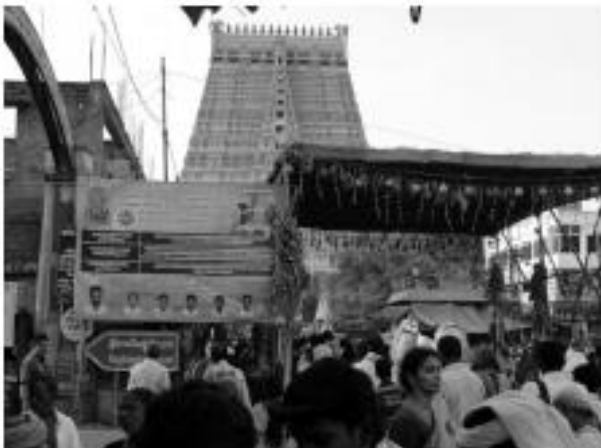
Figure: View of the Srirangam Rajagopuram hindered by assortment of components
