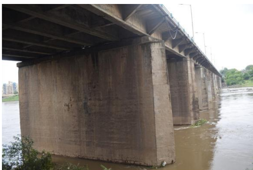
Image-(a): General view of Mundhwa Bridge across Mula-Mutha river
