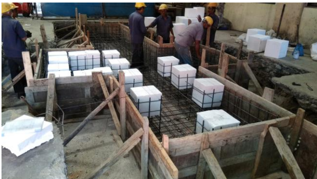
Fig 1. Use of Thermocole box as pockets formwork
