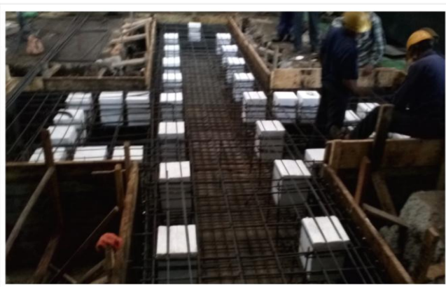
Fig 2. Thermocole box are aligned as per pockets of Machine
