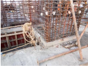
Column Starter Concrete
