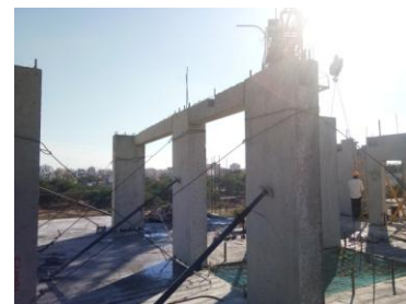
Column Beam Erection
