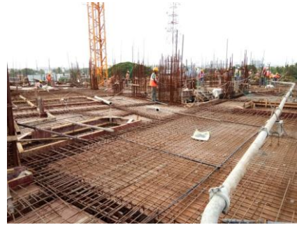
Slab Shuttering / Reinforcement
