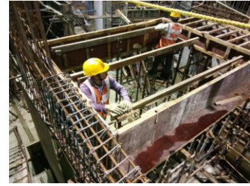
Beam Side Shuttering
