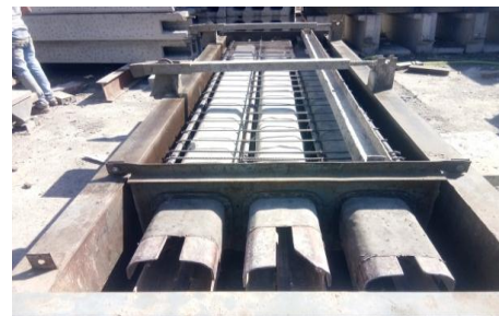
Column Mould with Reinforcement
