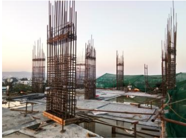
Column Starter Shuttering / Reinforcement
