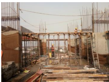
Beam Bottom Shuttering
