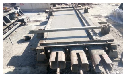
Pre-cast Column Concrete
