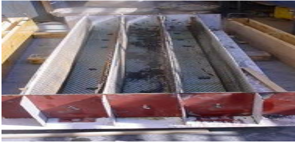
Figure 2. Mould for U-shape beam
