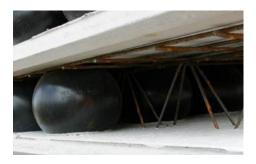
Bubble deck technology eliminates up to 35% of the structural concrete. When coupled with the reduced floor thickness and facade, smaller foundations and columns, construction costs can be reduced by as much as 10%. Using Bubble deck means floor cycles up to 20% faster than traditional construction methods.
