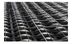
Construction: Depending on the manufacturer, plastic voided slab systems are constructed by two primary methods: a filigree method in which part of
