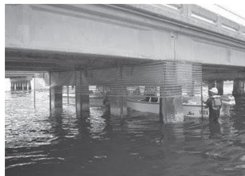
Fig 4.1 Mesh flooring around piles
