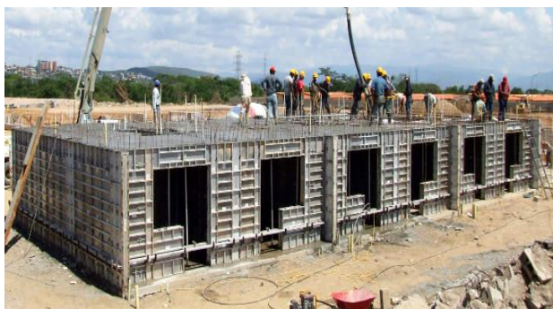
Aluminium Formwork Technology
