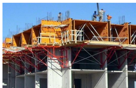
Tunnel Formwork Technology
