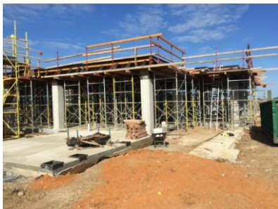
Conventional Formwork
