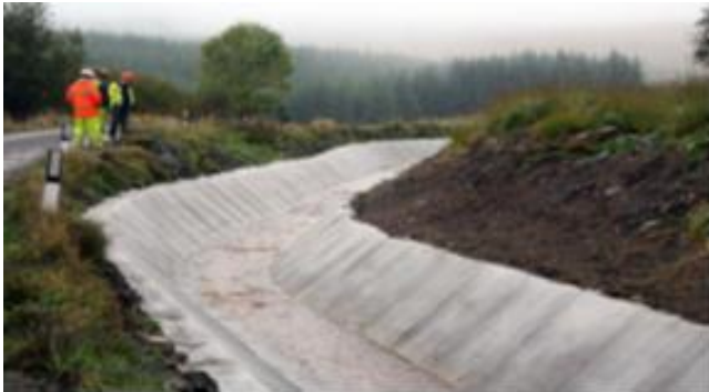
Figure 5:- Ditch lining [9]
