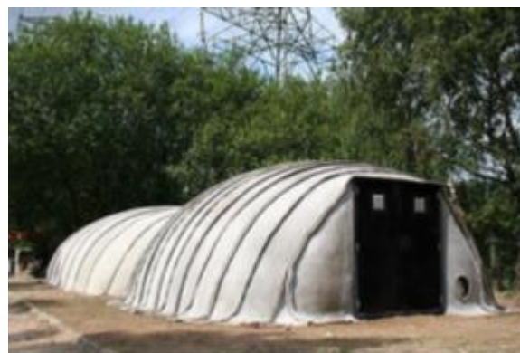
Figure 4:- Concrete Canvas Shelters [8]
