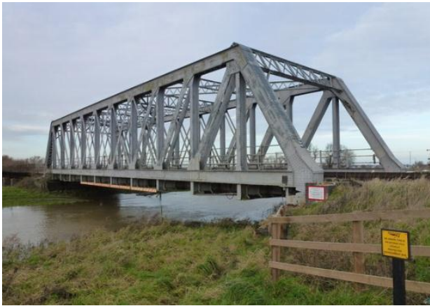
Fig .1 Truss Structure
