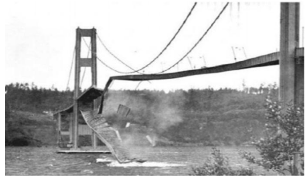
Fig .2 Bridge Collapse
