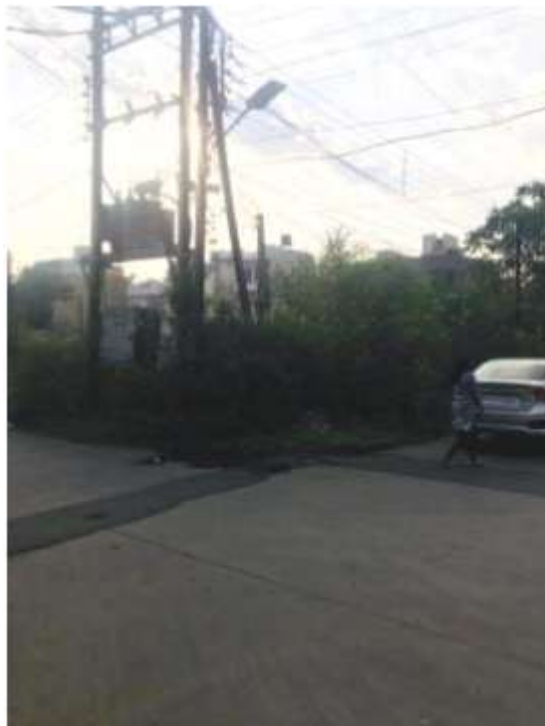
Figure 13 Dense vegetation; hiding places, obstructing views
