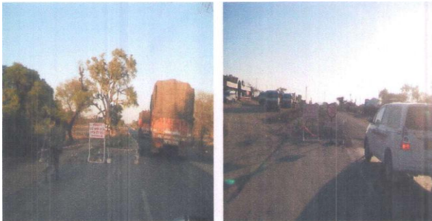
Approach transition zone is missing
