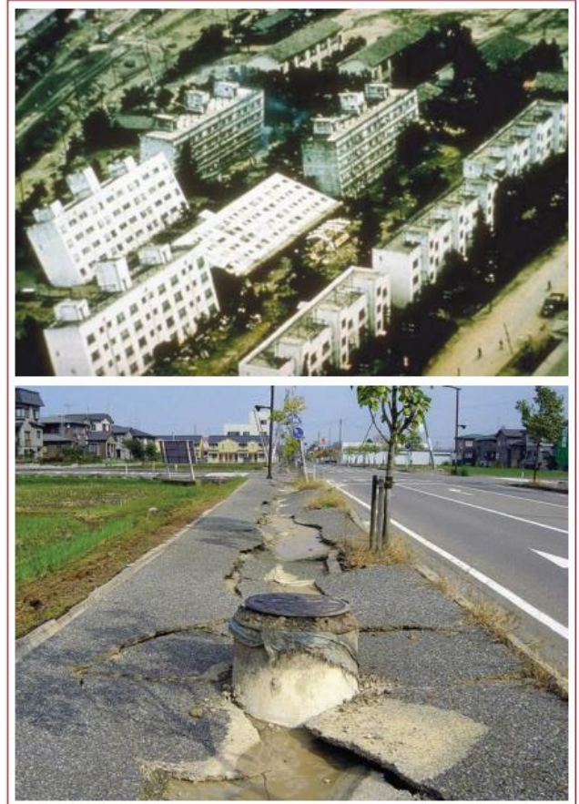
Figure 5: illustrates liquefaction-induced settling of flat buildings in Nigata, Japan, following the Earthquake of 1964 (courtesy of the University of Washington). The bottom photo shows one of the numerous manholes that floated to the surface in Nigata, Japan, as a consequence of the 2004 Chuetsu earthquake (photo courtesy of Wikimedia Commons).
