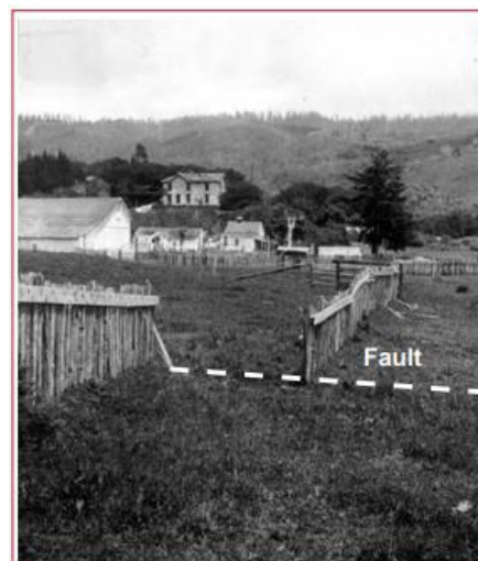
Figure 2: Fault movements can damage buildings and other structures by breaking the ground surface. When the San Andreas Fault
