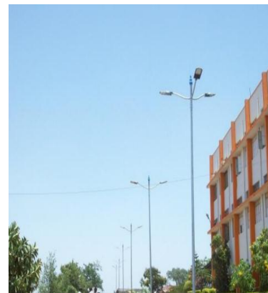
Fig.3.Street lighting near office building of campus
