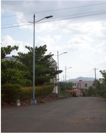
Fig.4. Street lighting near boys hostel of campus
