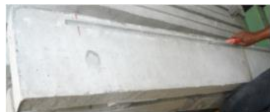
(a) Groove cleaning by high pressure air jet
