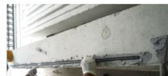
(c) Strengthening bar inserting
