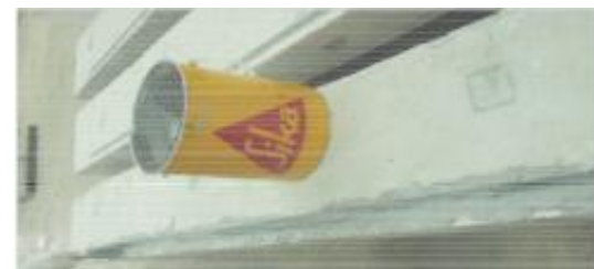
(b) Groove half fill using epoxy adhesive
