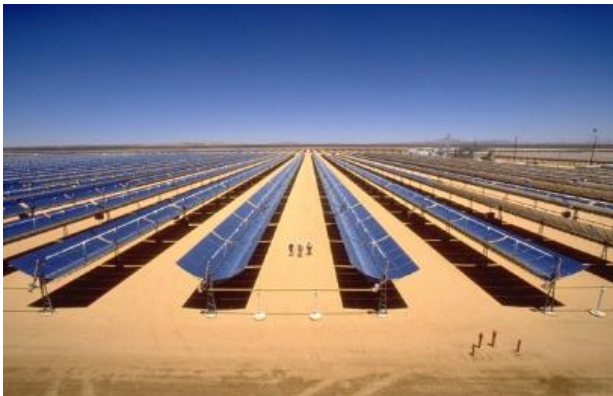
Fig. 1: Parabolic Solar Trough System at Kramer Junction, Mojave Desert, California
