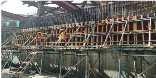
Fig. 1.4: Correct Alignment of Formwork
