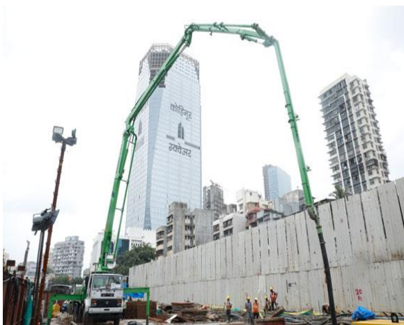
Fig 1.1: Use of Modern Equipment- Boom placer
