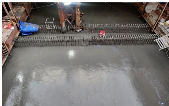
Fig. 1.5: Proper Levelling and Finishing by Skilled Meson
