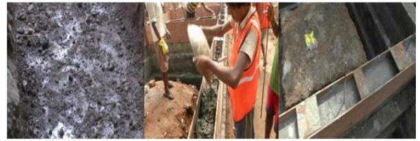
Figure 6: Foundation part of the construction
