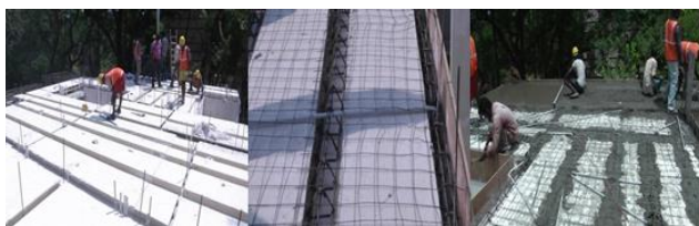
Figure 8: Roof slab construction
