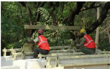
Figure 5: Transportation and lifting of the GFRG panel
