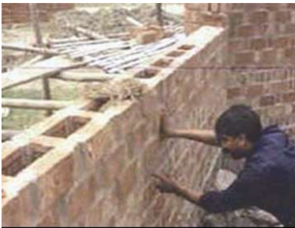
Fig. No 5 Rat trap Brick Masonry
