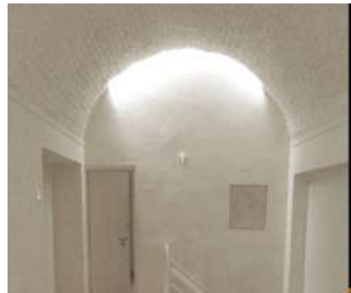
Fig. No. 7 after finishing
