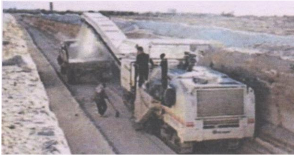
Trenching by surface miner
