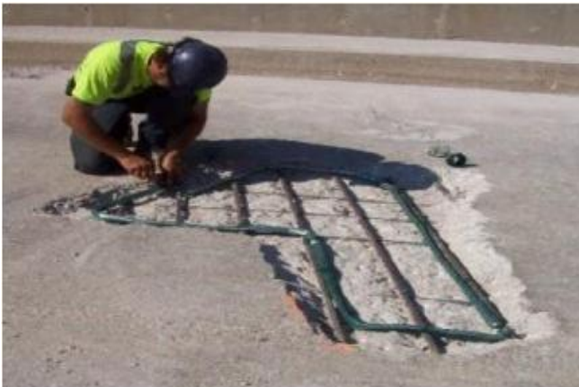
Figure 3. Shows the surface preparation of repairs
