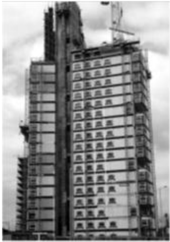
Fig1.25-storey modular building in Wolverhampton, England during construction (source:-By R. M. Lawson)
