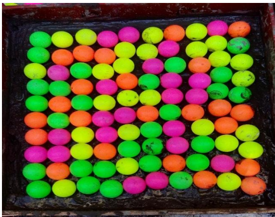
Fig. 2 Balls (bubbles) placed continuously over the reinforcement in grid form.
