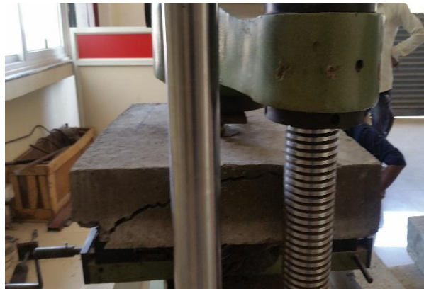
Fig.5 Crack patterns in Conventional slab.
