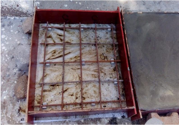
Fig 1 Reinforcement of conventional slab.
